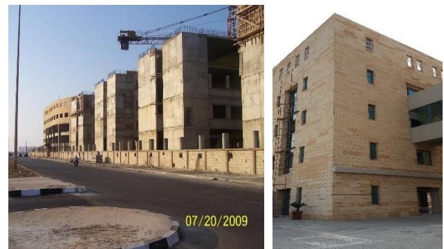
Figure 4: BAU campus under construction and stone cladding
