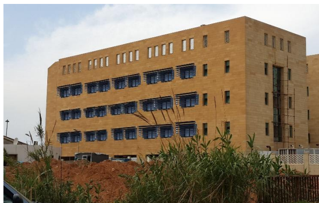
Figure 5. External shading devices proposed for south facade.
